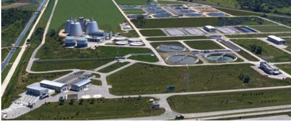
Fig. 2: Conventional wastewater treatment plant in Zagreb, Croatia
