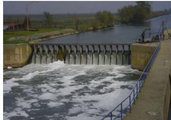
Fig. 4: Weir in Klek seen from downstream
