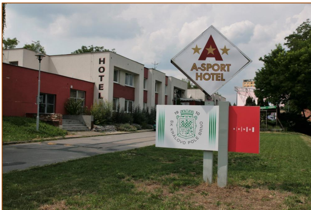
Hotel A-sport, Vodova 108, Brno-Královo Pole
