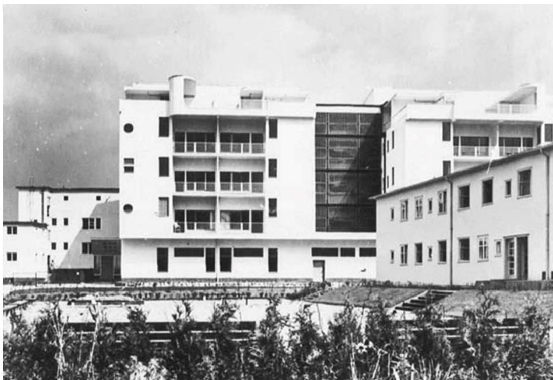
Fig.2: Photograph published in the "Moderner Wohnbau" journal in 1929. In the foreground is the common recreational area of the housing estate in the form of an immersed courtyard designed by Erich Vergin. In the background is model house No. 7 seen from the west and on the right side is multi-staircase tenement house No. 3-6
