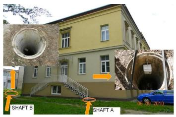
Fig. 2: Location of infiltration shafts near building PK6
