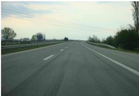
Fig. 13: More evident ruts on climb
