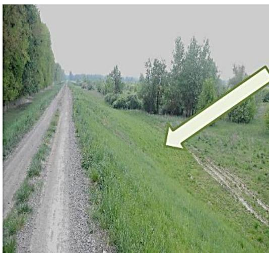
*Fig. 3: Disturbance of the levee on downstream face*
