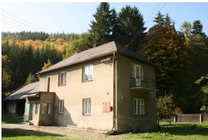
Fig.1: Residential building (south-east view)
