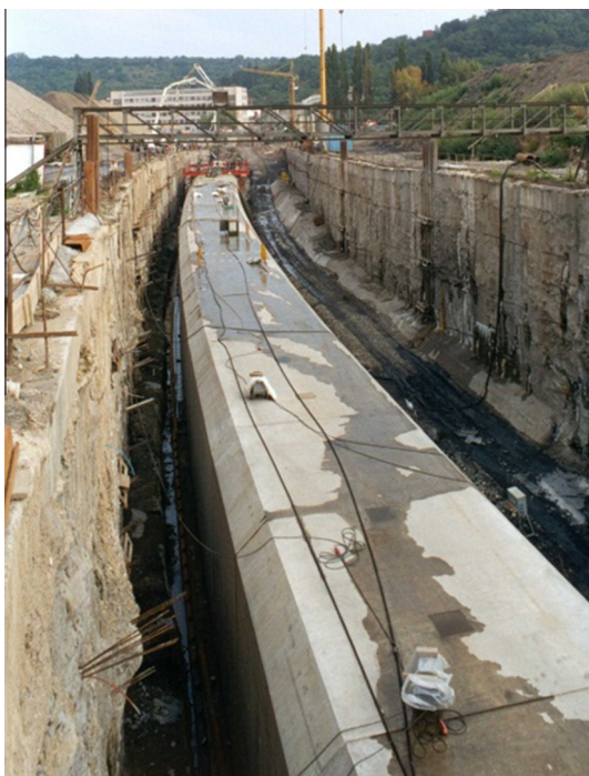
Fig. 12. A subway tube in dry dock.
