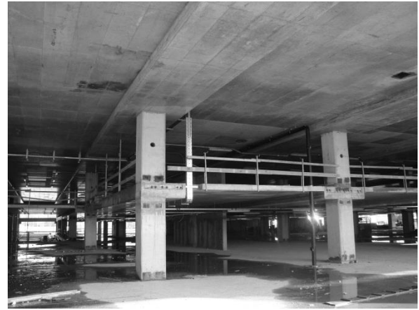
Fig. 5) Free tendon layout and inserted parking slab between two levels (8 by 16 m),
