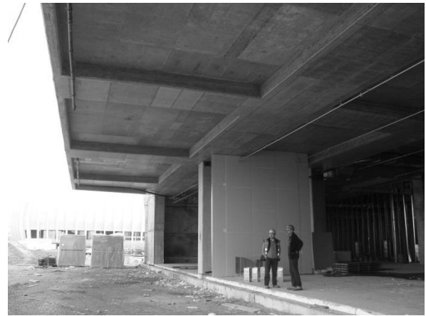
Fig. 6) 6.9 long cantilever used as a restaurant terrace
