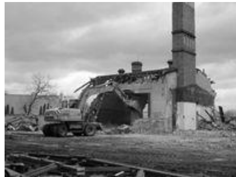
b) demolitions through the mechanization
