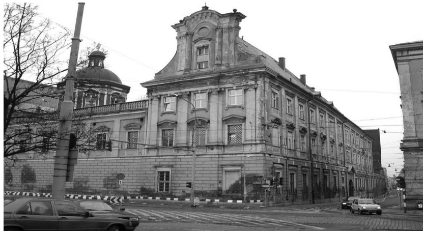
Fig. 2) View of building from south-western side before renovation (in 1999).
