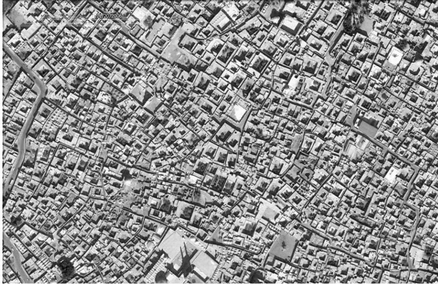
Fig. 2) Pedestrian walkway structure in Fahadan – Yazd [8]
