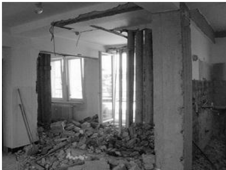
a) manually demolition of structures
