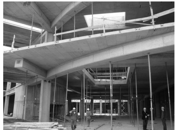
Fig. 7) Concreting of 16 by 16 m grid market, complex area zone of 18.5 m curved beam
