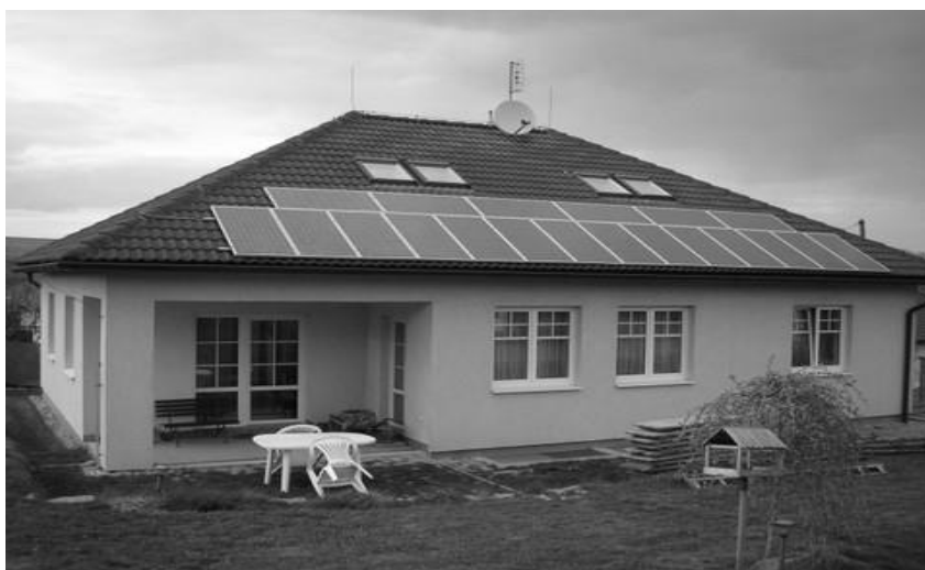
Fig. 1) Solar power photovoltaic panels on the roof of a house [8]
