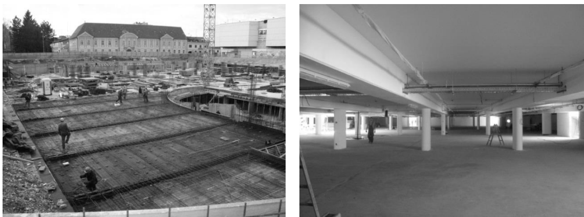
Fig. 9) Constructing and arranging of underground garage interior
