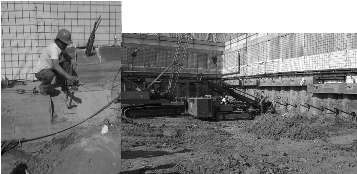
Fig. 2) & 3) Construction pit protection
