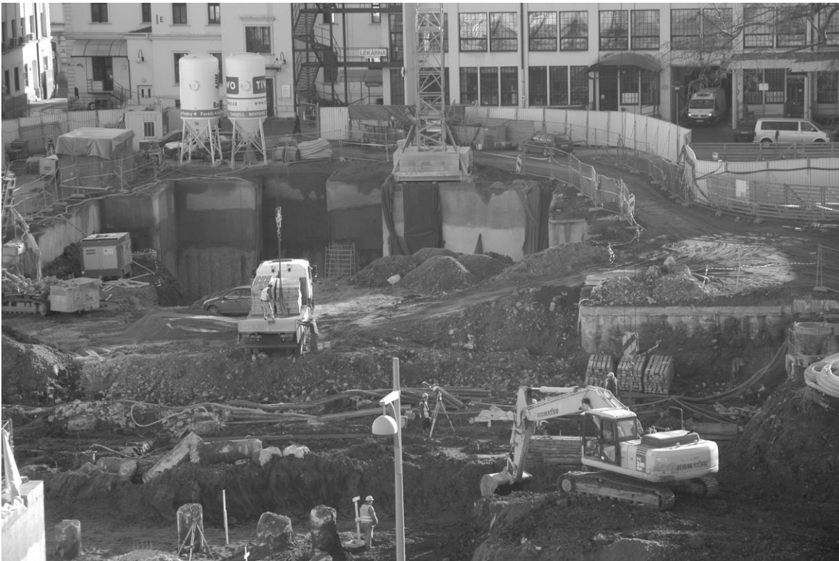
Fig. 3) Special foundation – underground walls of ICRC basement
