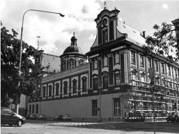
Fig. 13) View of building from north-western side after renovation.
