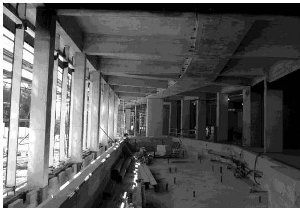
Fig. 10) Indoor swimming pool construction
