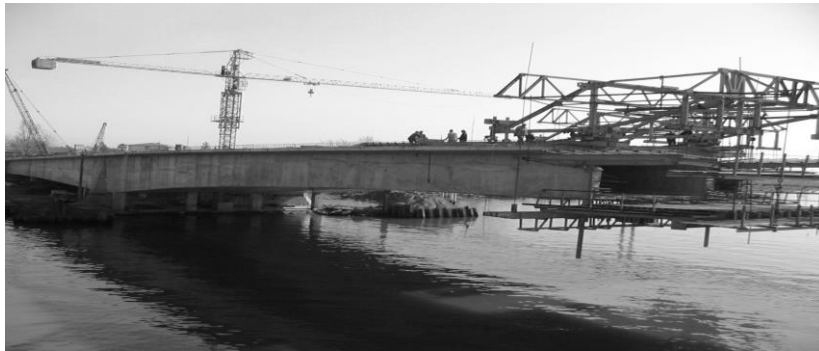
Fig. 2) Box bridge implemented by balanced cantilever method (Photo by J. Razzaghi)
