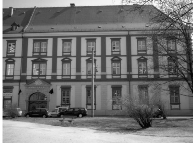
Fig. 14) View of building's west facade in 2012.
