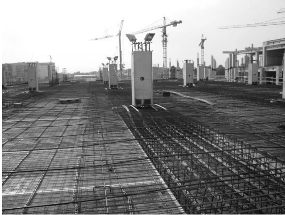
Fig. 5) Free tendon layout and inserted parking slab between two levels (8 by 16 m),
