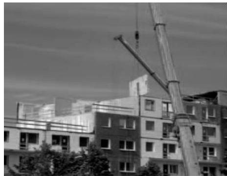
d) deconstruction of structures
