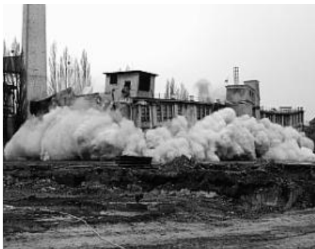
c) demolition of construction by explosion
