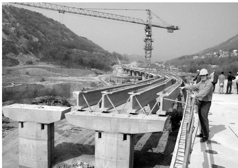
Fig. 5) Precast concrete bridge construction
