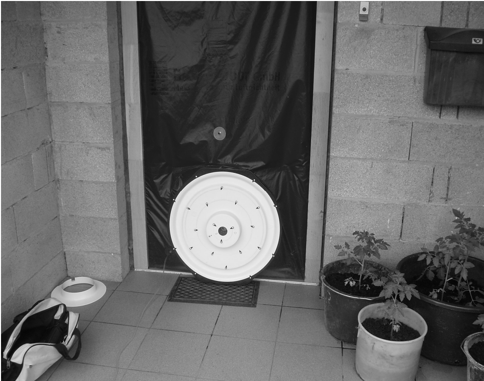
Fig. 1) Measurement of the building envelope air-tightness
