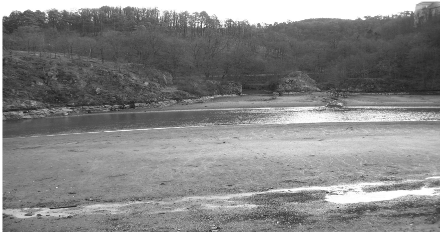
Fig. 4) The sediment on the reservoir bottom appears when the level of water is reduced
