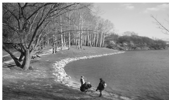
Fig. 1) Bank stabilization – Brno damm (foto M.Šlezinger, 2008)
