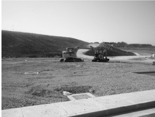
Fig. 5) Kaštijun landfill during remediation
