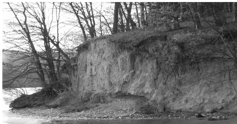
Fig. 3) An example of abrasive damage to the Brno Reservoir banks
