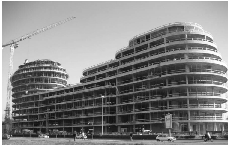
Fig. 1) Construction of residential – office building ACC
