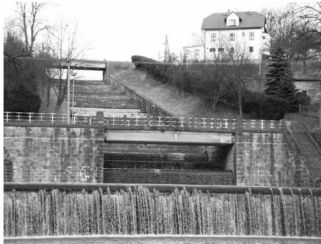
Fig. 1) Upstream view on stepped spillway of the Bystřička dam (taken by Povodí Moravy, s.p.).
