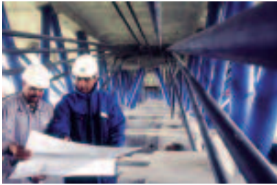
Boulonnais Viaduct, France - 1996
