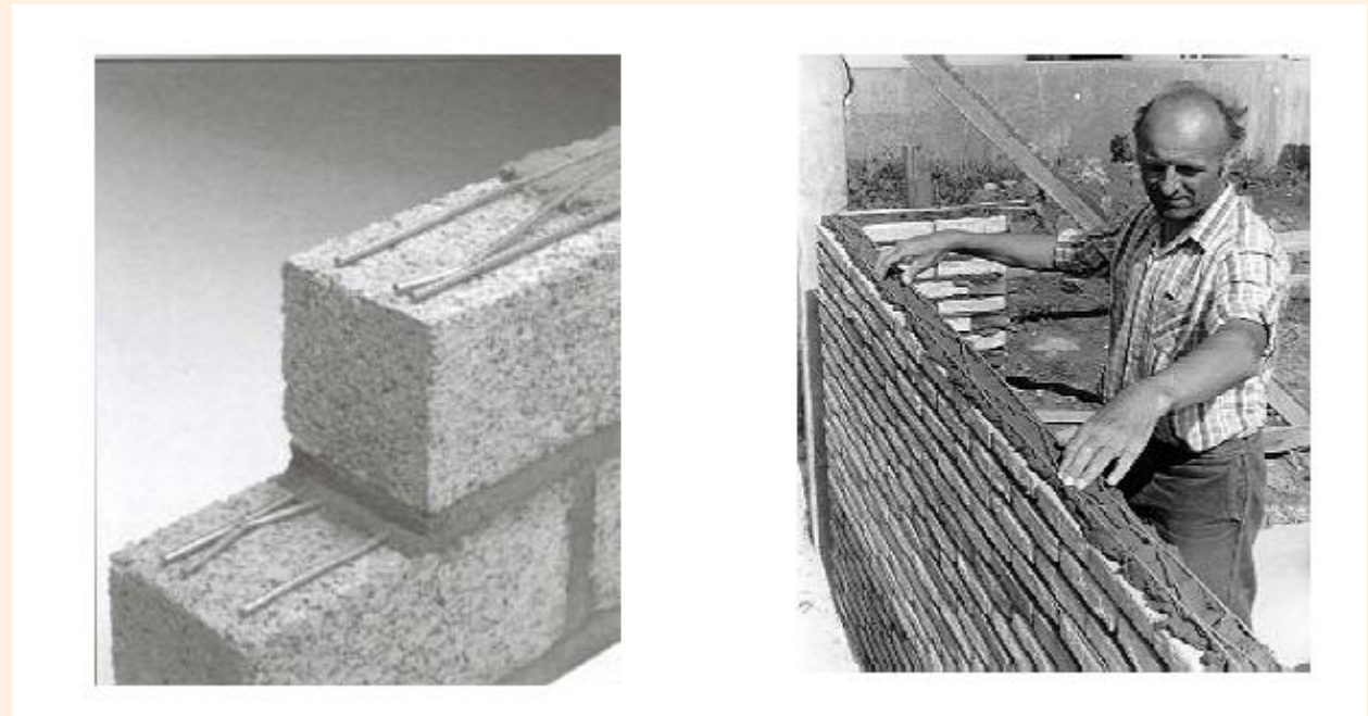
Masonry wall horizontal joint reinforcement
