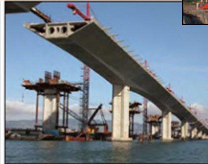
Use of prefabricated segmental construction is one way to accelerate bridge construction. Here, hinge pipe beams at mid-span expansion joints are being incorporated in the San Francisco - Oakland Bay Bridge
