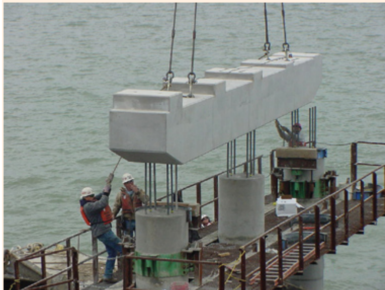
Use of prefabricated segmental construction is one way to accelerate bridge construction. Here, hinge pipe beams at mid-span expansion joints are being incorporated in the San Francisco - Oakland Bay Bridge
