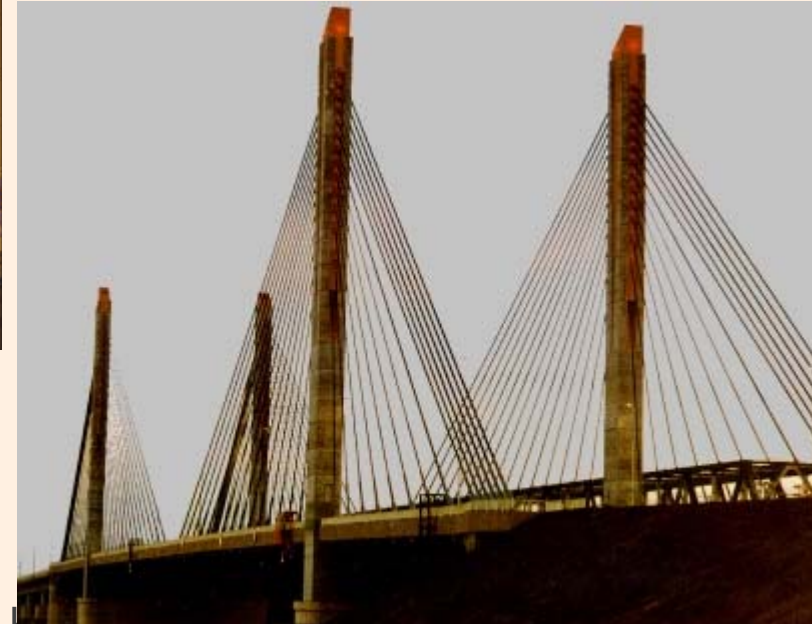
Crosses the river Waal south-east of Rotterdam, Netherlands
