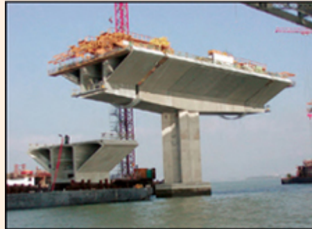
Use of prefabricated segmental construction is one way to accelerate bridge construction. Here, hinge pipe beams at mid-span expansion joints are being incorporated in the San Francisco - Oakland Bay Bridge
