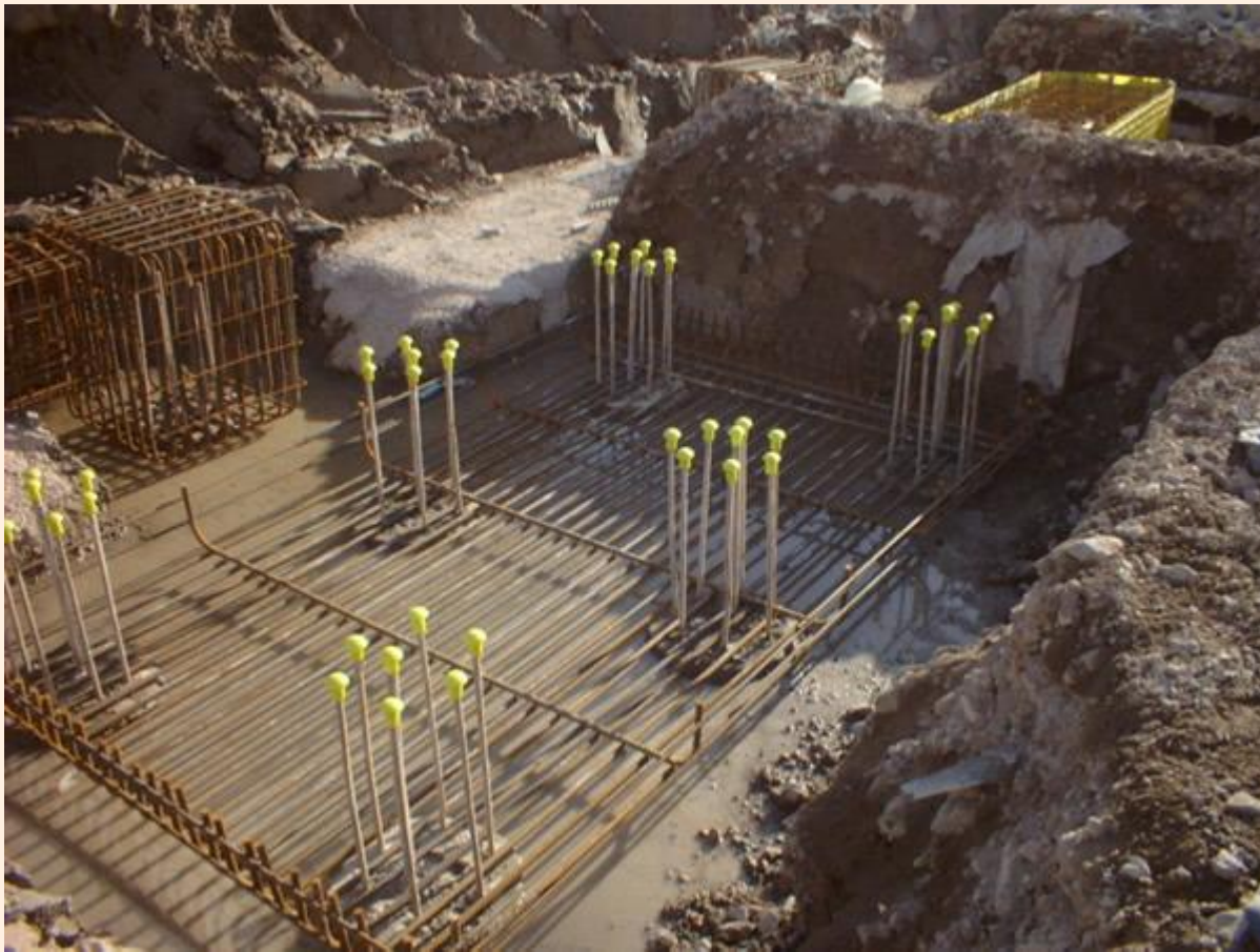
Preformed bottom cage of reinforced ground beam set over 6 piles
