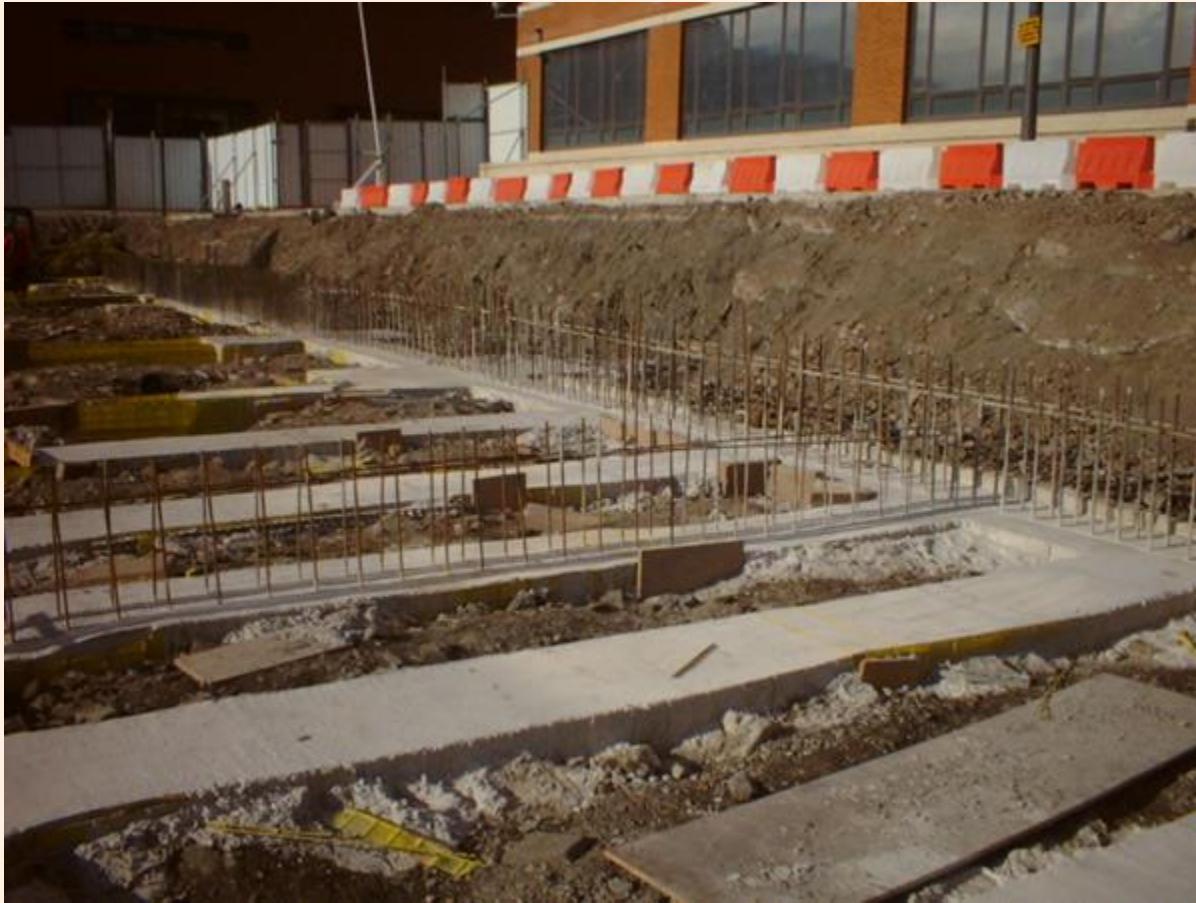
Ground Beams for the Stair Tower and Bridge Links
